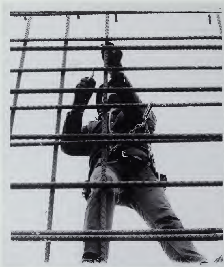
Fig. 2-26. Tying rebar—construction began on the nuclear hardened facilities in 1970.
